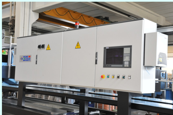
Main Electric control board
